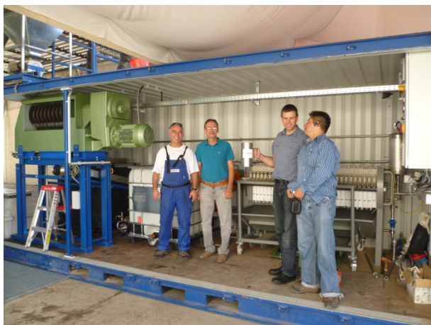
Fig. 14 CompacTropa oil mill in Manabi.
