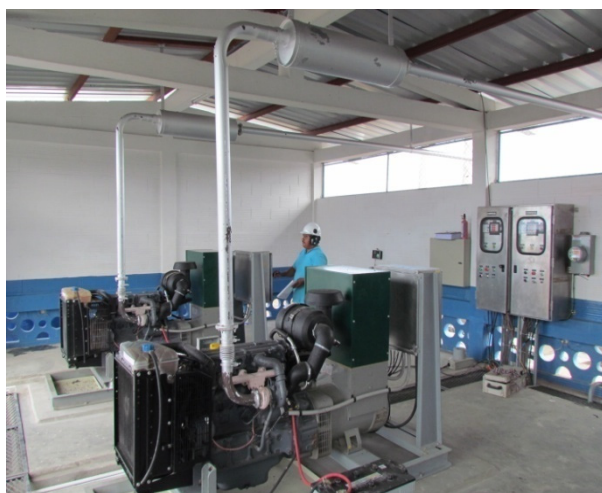
Fig. 11 Jatropha gen-sets 2 × 69 kW el. on Floreana.
